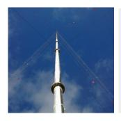
**SLX1/W:**GUYED TUBULAR TEMPORARY MET MAST TO 70M
